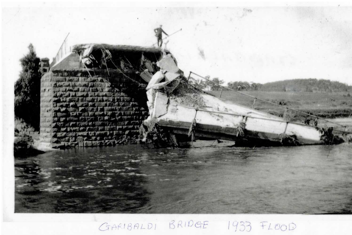
Image 47: Photograph of the Garibaldi Bridge Flood in 1933.
